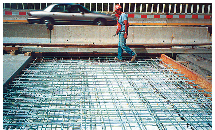
Galvanized rebar offers economical long term protection before and after installation.
